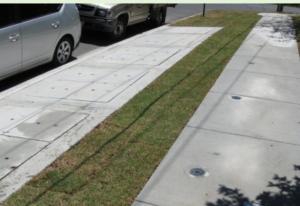
OdaVent® MHV installed in a street verge - St Lucia, Qld
