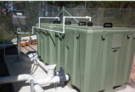
The OdaVent® MHV can be installed above or below-ground.
